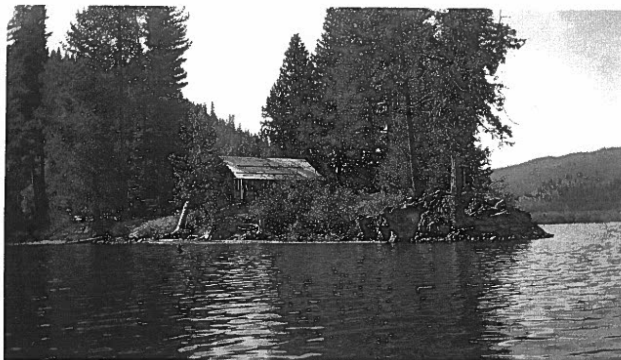
ELVIN BITO BUILDING NEW CABIN AT POINT, HEAD OF SPIRIT LAKE, EARLY 1950'S
