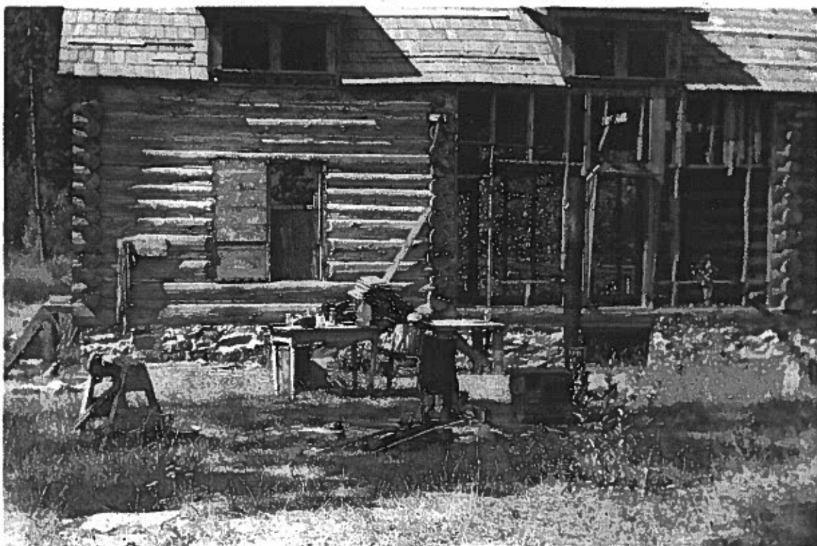
ELVIN BAITO TEARING DOWN JENKINS LODGE Ruined By Wood Cutters During WWII LATE 1940'S
