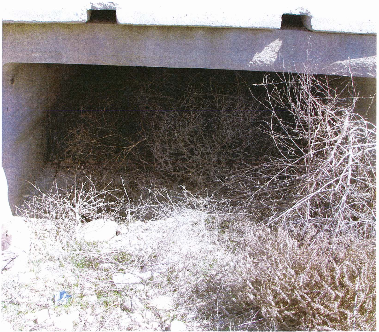
West side looking under Bridge.
