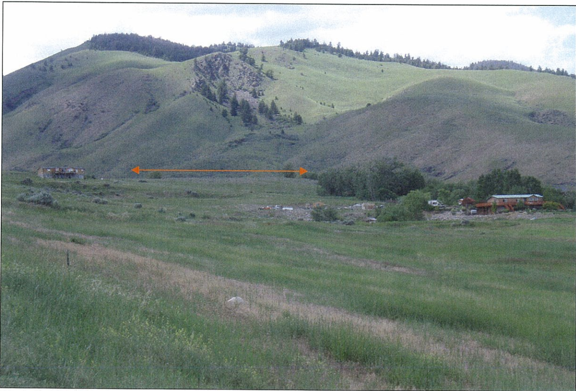
Photo 9 (6/25/09) - Embankment from a downstream vantage point. The crest is highlighted with a colored line stretched above its length. In foreground is the small pond (shown above).
