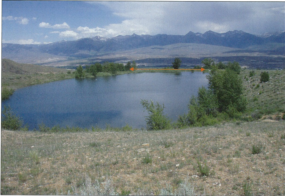
Figure 7 (6/25/09) - Overview of existing dam (background) and reservoir. The treed area in the photograph right-front corner is the channel carrying water from the spring to the reservoir.
