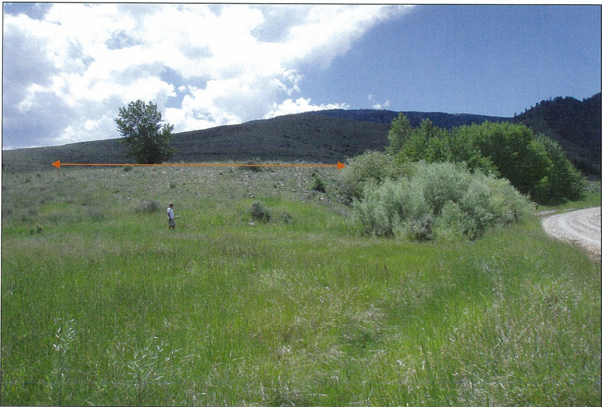
Photo 5 (6/25/09) - View looking at the downstream slope of the dam near maximum section. Note the location of Oliver Road (right), and the heavy growth of vegetation on north side of the embankment.
