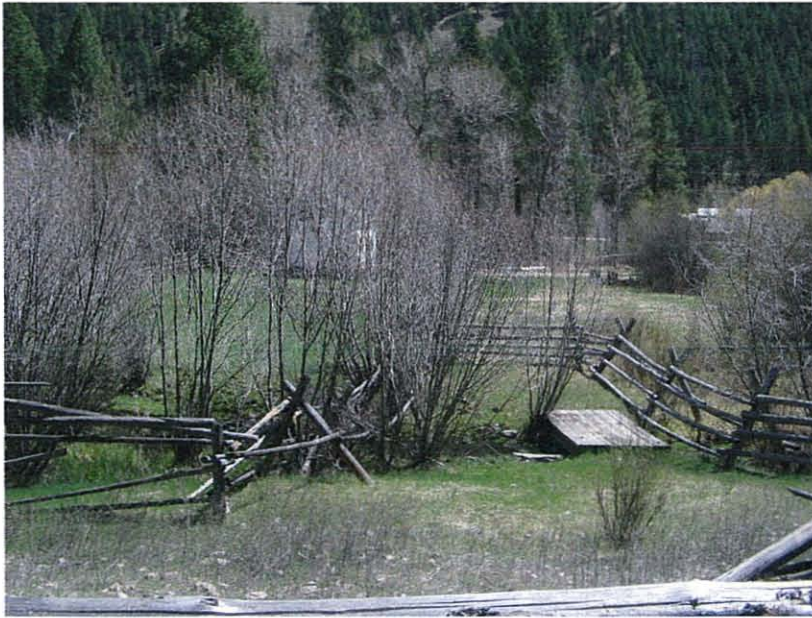
An overland view of the footbridge. The channel enters the land from the left and flow direction is to the right. The footbridge is clearly seen in the right third of the picture.
