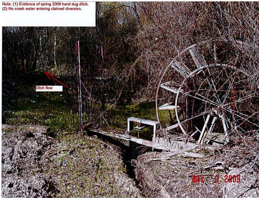
PHOTO 1458; (1) No creek water entering abandoned fish screen. (2) The photo illustrates that the creek water enters from the close side and the ditch flow is in the direction of the arrow. (3) Pile of sod and earth is evidence of the recently dug ditch.
