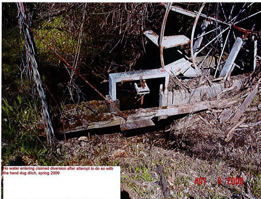
PHOTO 1457; Hand dug ditch with no creek water entering the abandoned fish screen.
