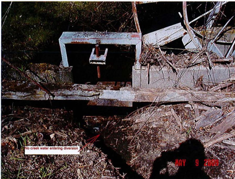
PHOTO 1462; Depicts no creek water entering the abandoned fish screen structure from the incoming (Carmen Creek) side. The water on the back side of the concrete wall is a collection of spring and waste water.
