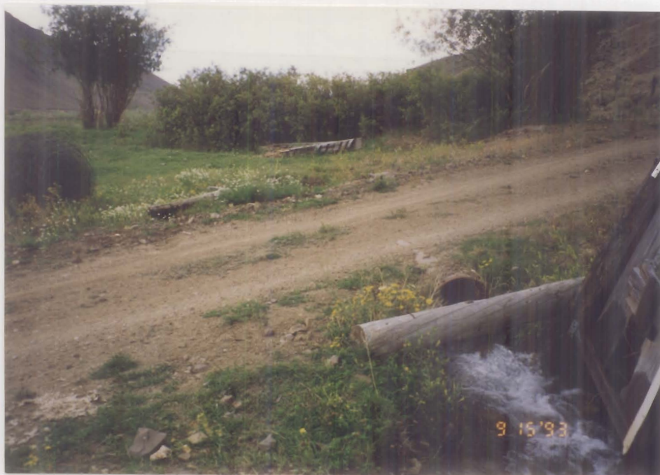
SHERWOOD ditch as it goes along the west side of prop- erty and continues North to INGRAM.
