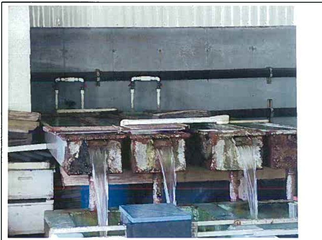
Photo 8. Looking in a southerly direction at the water coming into the small raceways. The supply line is 1-inch PVC pipe that dumps water into the trough then it flows into the small raceways. A 4-inch pipe from Spring Creek supplies the hatchery water.
