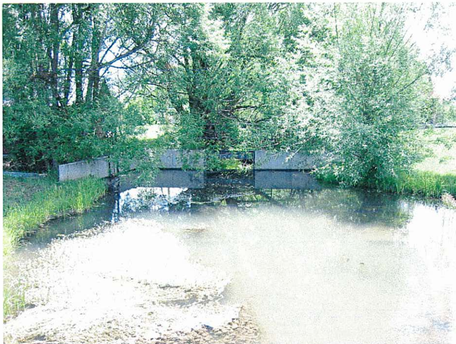
Inlet to headgate (tag Ao008782) viewing east.
