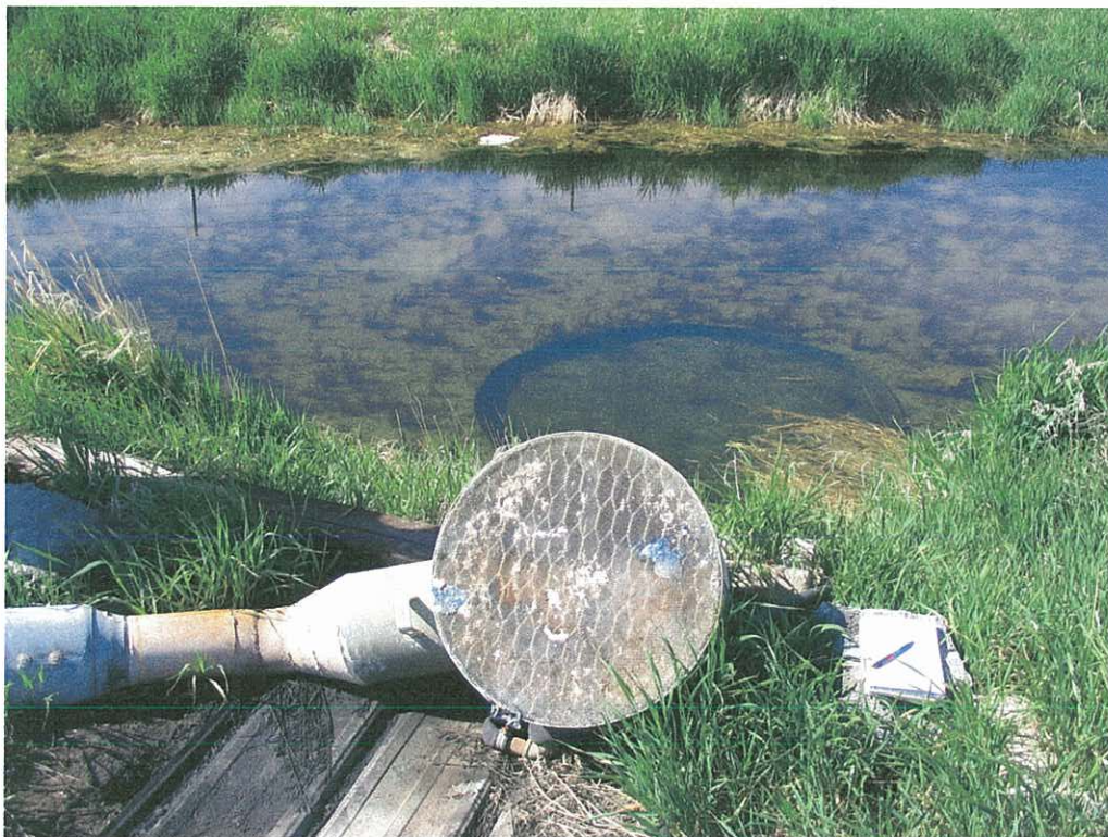
A22-13463 pump station location, looking South.
