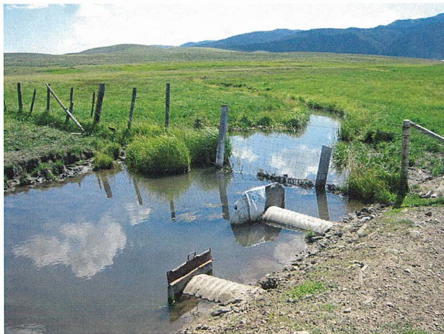
POD from section 33 and view is southwest.
