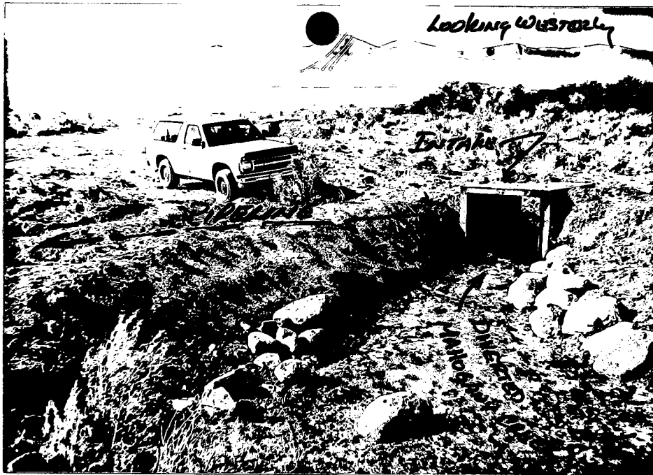
Photo 2c. NEW MAHOGANY CK INTAKE TO NEW PIPELINE. THIS IS NOT THE ACTUAL POINT OF DIVERSION, ALTHOUGH, THE TWO MAY HAVE THE SAME LEGAL.
