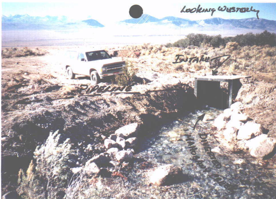
Photo 2c. NEW MAHOGANY CK INTAKE TO NEW PIPELINE. THIS IS NOT THE ACTUAL POINT OF DIVERSION, ALTHOUGH, THE TWO MAY HAVE THE SAME LEGAL.
