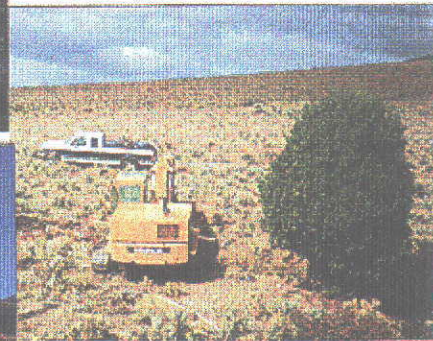
DITCH CLEANING NEAR MAGPIE SPRINGS.
