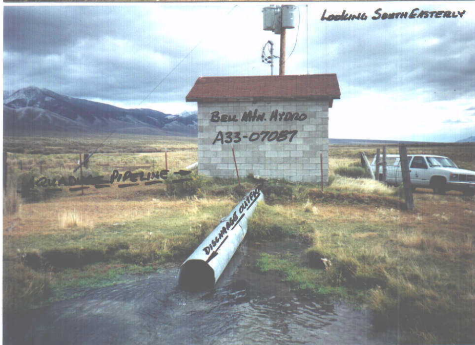
Photo 9b. View of BELL MTN. HYDROPLANT Looking SOUTH-EASTERLY.
