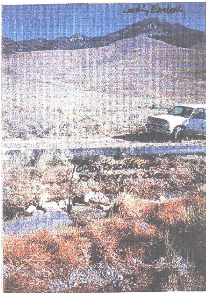
Photo 2d. SHOWS OPEN DISCHARGE OF NEW PIPELINE TO EXISTING DITCH AT SENEBW SEC. 30 T.11N., R. 27E.
