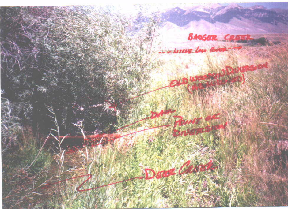
Photo 1. POINT OF DIVERSION FROM DEER CREEK. SHOWS PRESENT AND OLD POINT OF DIVERSION WORKS
