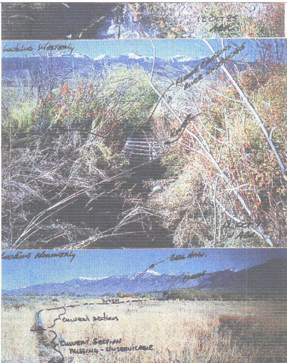
Photo 2. OLD UNSERVICABLE FLUME CROSSING LITTLE Lost RIVER (HIDDEN IN UNDERGROWTH-FLOWING RIGHT TO LEFT). THIS FLUME CARRIED BADGER CREEK AND/OR LITTLE Lost RIVER EXCHANGE WATER TO THE WEST SIDE OF LITTLE Lost RIVER. SEE DEER CREEK CLAIM A33-10119. NO LONGER USED.
