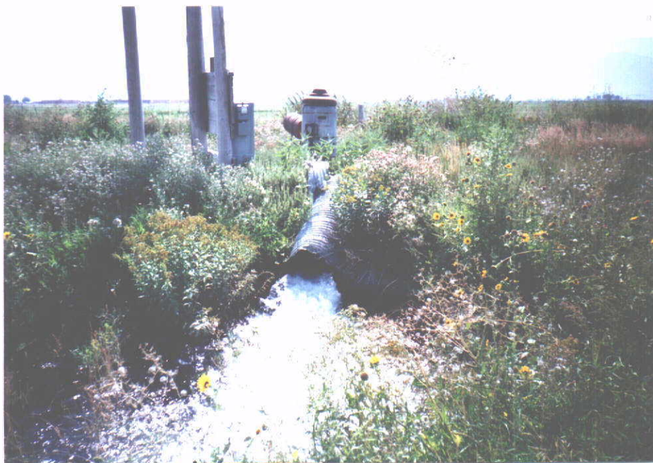
Photo 3. DISCHARGES TO OPEN
