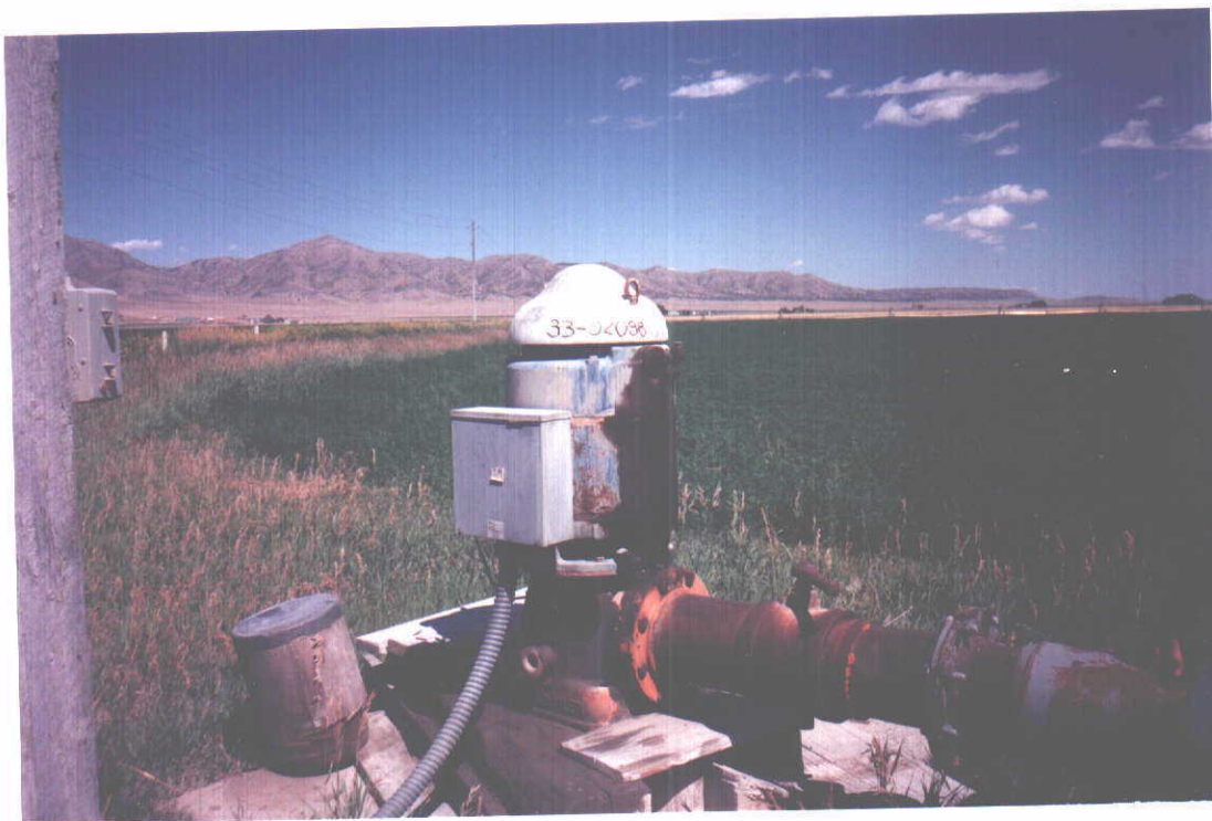
* Well at NWNWSW, S23, T6N, R29E. Photo faces east.
