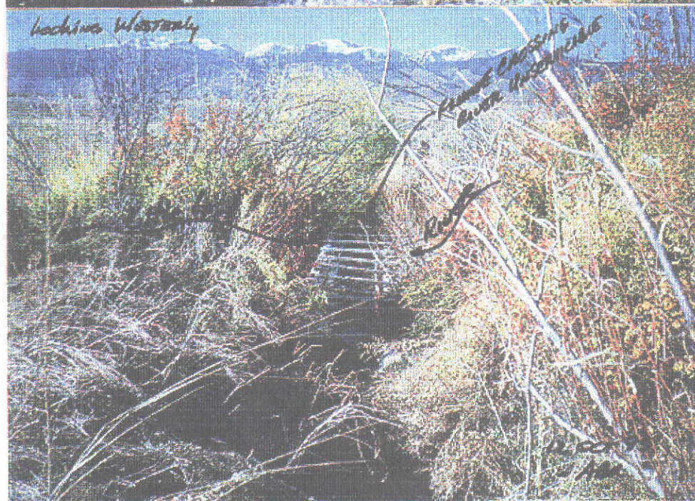
Photo 2. OLD UNSERVICEABLE FLUME CROSSING LITTLE LOST RIVER (HIDDEN IN UNDERGROWTH - FLOWING RIGHT TO LEFT). THIS FLUME CARRIED BADGER CREEK AND/OR LITTLE LOST RIVER EXCHANGE WATER TO THE WEST SIDE OF LITTLE LOST RIVER. SEE DEER CREEK CLAIM A33-10119. NO LONGER USED.
