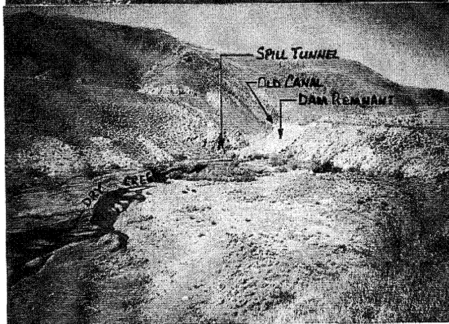
Photo 3. OLD DRY CREEK DAM WHICH IS REFERENCED IN THE DECREE AS THE POINT OF DIVERSION FOR THE DRY CREEK RIGHTS. THIS DAM WAS BLOWN IN THE 1930'S BUT DID NOT FAIL UNTIL 1956. IT WAS BLOWN DUE TO A WATER FIGHT BETWEEN THE OLD SETTLERS AND THE BLAINE COUNTY INVEST. Co. ALL PHOTOS LOOKING NORTHERLY. PHOTOS TAKEN: 31 Oct. 95 ABR
