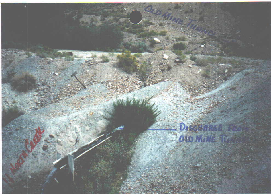
Photo 1. Shows the DRAINAGE FROM THE OLD MINE TUNNEL INTO NORTH CREEK. MAKES UP ABOUT \frac{1}{2} OF THE CREEK FLOW.
