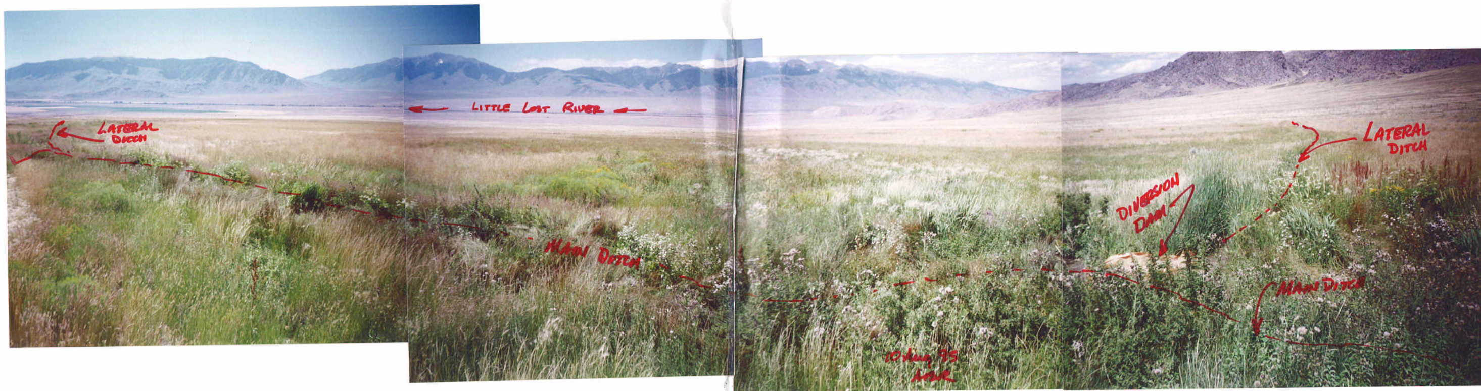
Photo SET. SHOWING LATERAL DITCH WITH CANVAS DAM DIVERSION, ONE OF SEVERAL DITCHES USED TO FLOOD IRRIGATE WESTSIDE OF THE MAIN DITCH. SEE ASCS PHOTO COPY FOR LOCATION.
