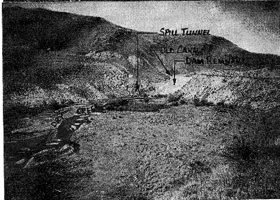
Photo 3. OLD DRY CREEK DAM WHICH IS REFERENCED IN THE DECREE AS THE POINT OF DIVERSION FOR THE DRY CREEK RIGHTS. THIS DAM WAS BLOWN IN THE 1930'S BUT DID NOT FAIL UNTIL 1958. IT WAS BLOWN DUE TO A WATER FIGHT BETWEEN THE OLD SETTLERS AND THE BLAINE COUNTY INVEST. CO. ALL PHOTOS LOOKING NORTHERLY. PHOTOS TAKEN: 31 Oct. 95 ABR
