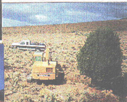
DITCH CLEANING NEAR MAGPIE SPRINGS.
