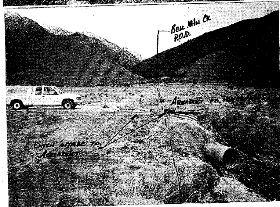
Photo 8. DITCH INTAKE TO AQUADUCT. BELL Mtn. CK IN BACKGROUND. NESESW SEC. 5 T. 10N, R. 27E.
