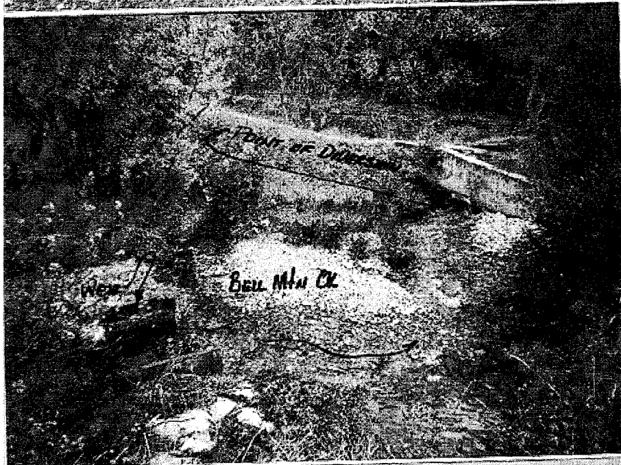
Photo 7. POINT OF DIVERSION OF BELL Mtn. CK TO HYDROPLANT AQUADUCT. SESENE SEC. 5 T. 10N, R. 27E.
