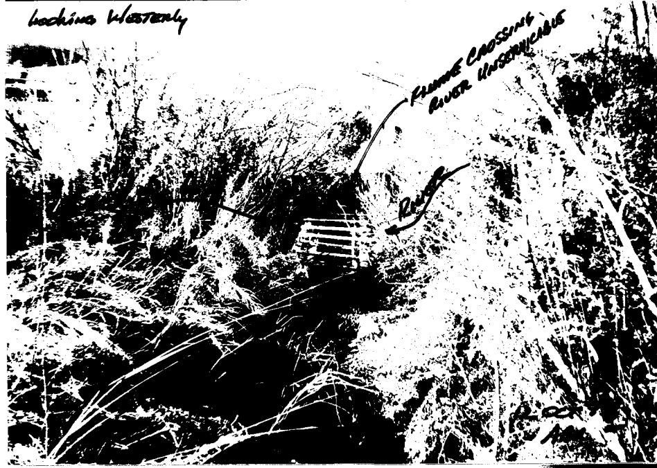
Photo 2. OLD UNSERVICABLE FLUME CROSSING LITTLE LOST RIVER (HIDDEN IN UNDERGROUNTH-FLOWING RIGHT TO LEFT). THIS FLUME CARRIED BADGER CREEK AND/OR LITTLE LOST RIVER EXCHANGE WATER TO THE WEST SIDE OF LITTLE LOST RIVER. SEE DEER CR CLAIM A33-10119. NO LONGER USED.
