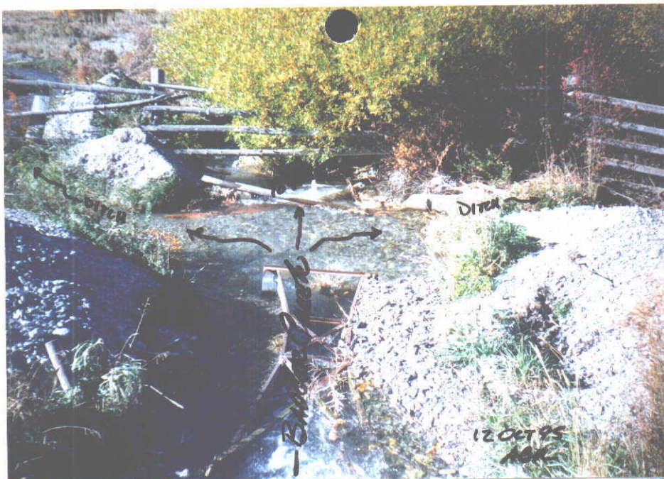
Photo 1. TAKEN FROM THE LITTLE LOST RIVER HIGHWAY AT THE BADGER CREEK CULVERT. THIS IS THE POINT OF DIVERSION FROM BADGER CR. AN EXCHANGE DIVERSION FROM THE LITTLE LOST RIVER IS ALSO USED (SEE PHOTO 4 THIS SET) USE OF BADGER CREEK WATER IS EXCHANGED FOR LITTLE LOST RIVER RIGHT 33-00032. (CLAIMED AS: A33-00032A).
