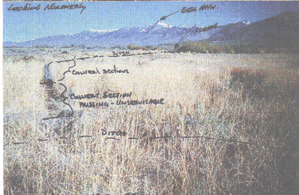
Photo 3. SHOWS THE OLD DITCH AND CULVERT SECTIONS WHICH ONCE CONVEYED BADGER CREEK WATER (A LITTLE LOST RIVER EXCHANGE WATER) TO THE AREA NOW CLAIMED AS SERVICED BY DEER CREEK WATER. SEE A33-10119.
