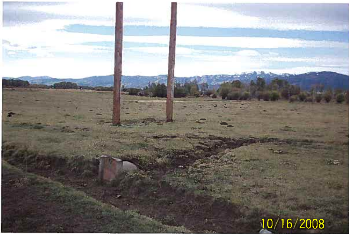
Photo 3 Delivery system southwest of the north pond.
