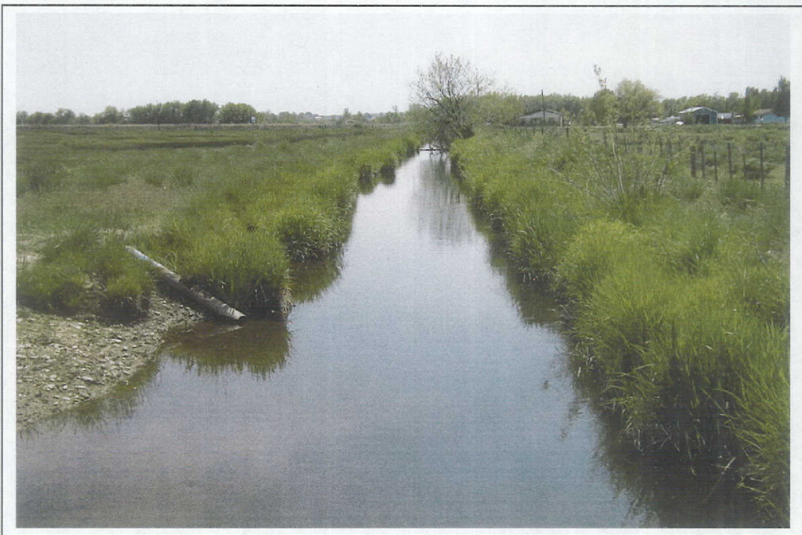
Colwell FX 5/15/03 Area 6: T08N, R04W, S35, NWNW, Johnson Higby Ditch. View to South.
