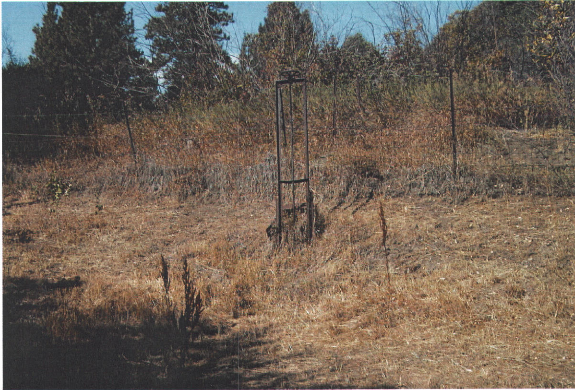
Photo 3. Field exam 8/31/01 photos by RDH. Outlet controls, overflow is put back into Smith Creek.
