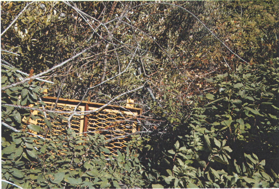
Photo 1. Field exam 8/31/01 photos by RDH. Back side of concrete culvert (18") from Smith Creek to pond. T02N, R07E, S13, SENWSW.
