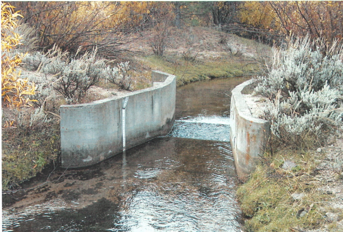
Photo 3: Weir, located in ditch just below POD. View is to South.
