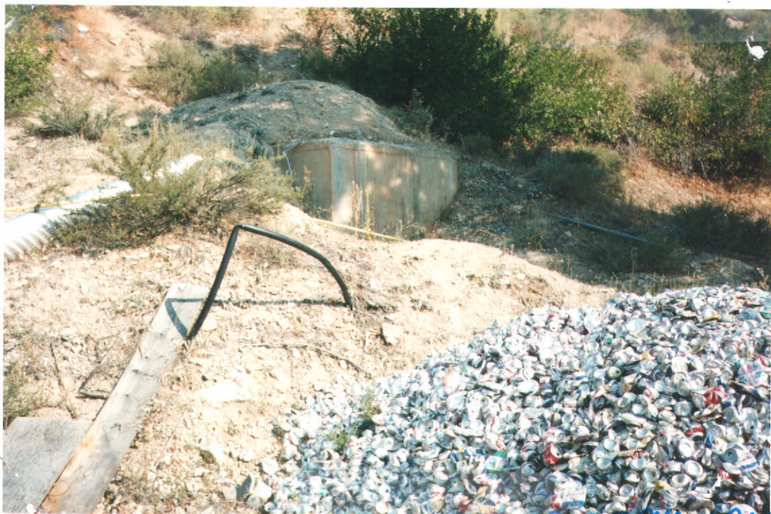
Holding tank for well water.
