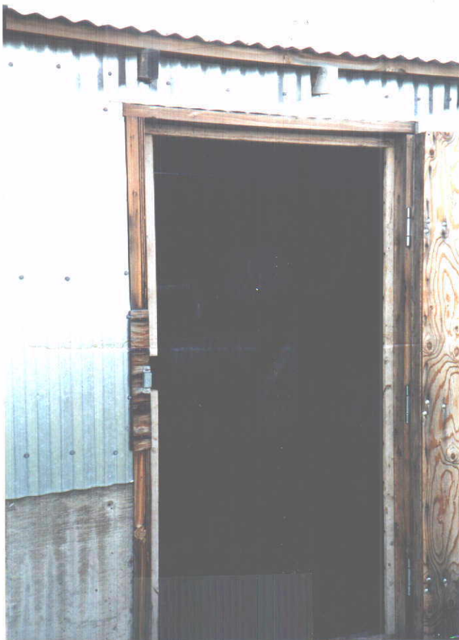
POWER GENERATOR - SMELTER GULCH SOURCE.
