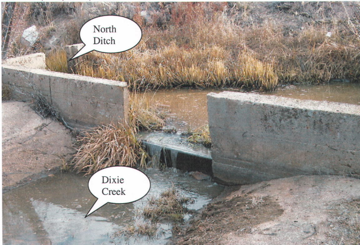
Photo 1. FX Nov.13, 2001. Photos by RDH. 63-00118A & B. Concrete dam located in the SENE, S23, T01S, R08E.
