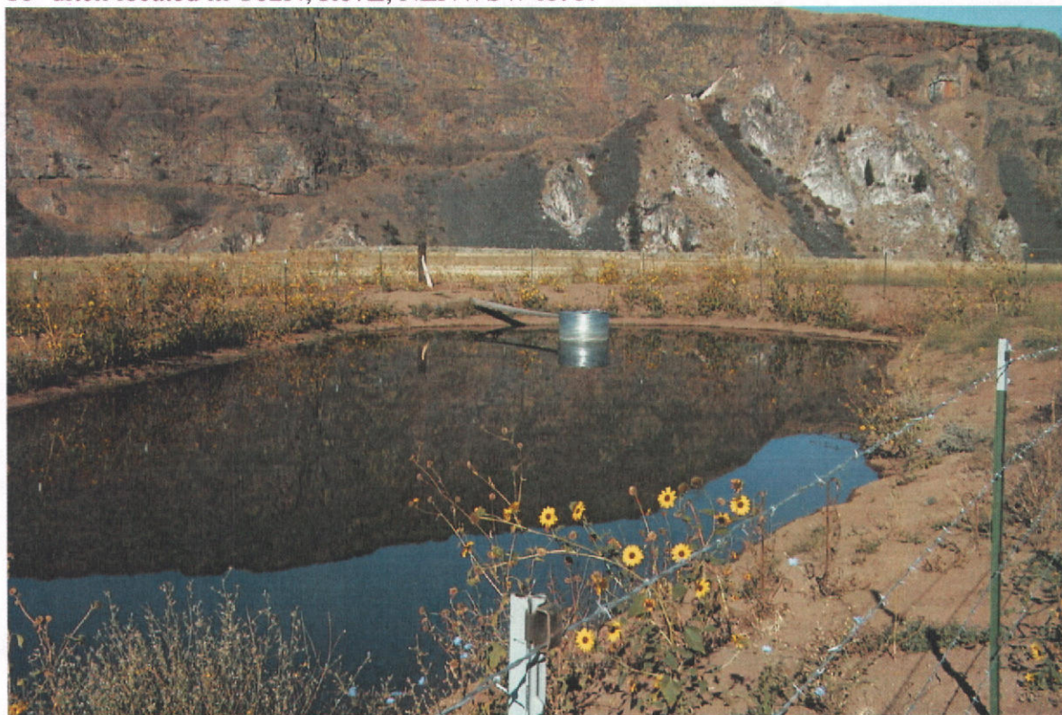
Photo 2. Distribution pond was built in 2000-2001 to improve on big ditch loss problem. Located in T02N, R06E, NWNW, lot 2.
