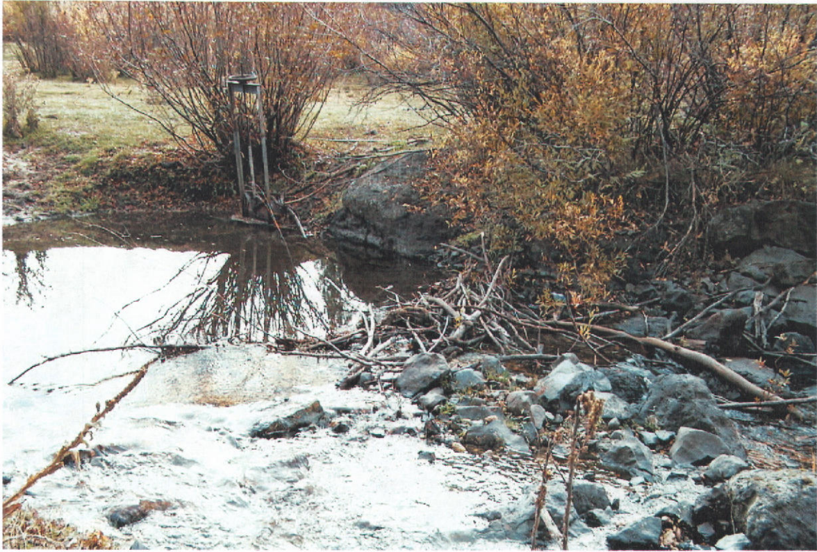
Photo 3: View shows rock dam and head gate from West bank to East side.
