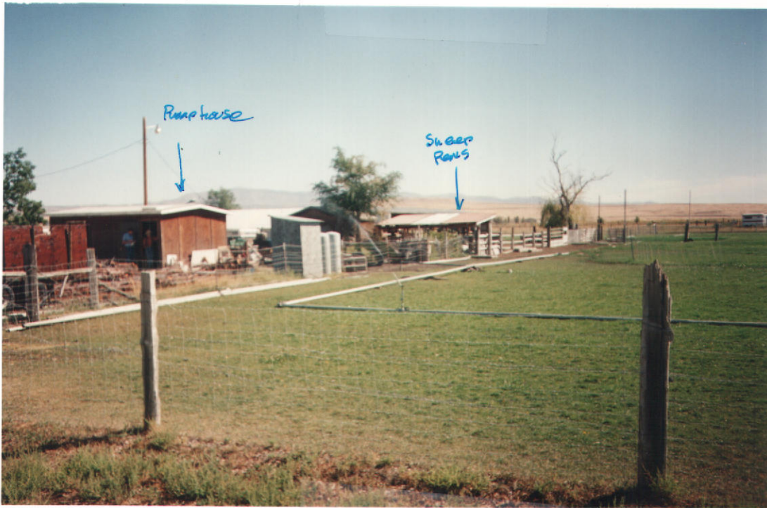
Photo #1-10 Looking East From West Side of Property Showing Part of Pasture, Pump house, Sheep Pens
