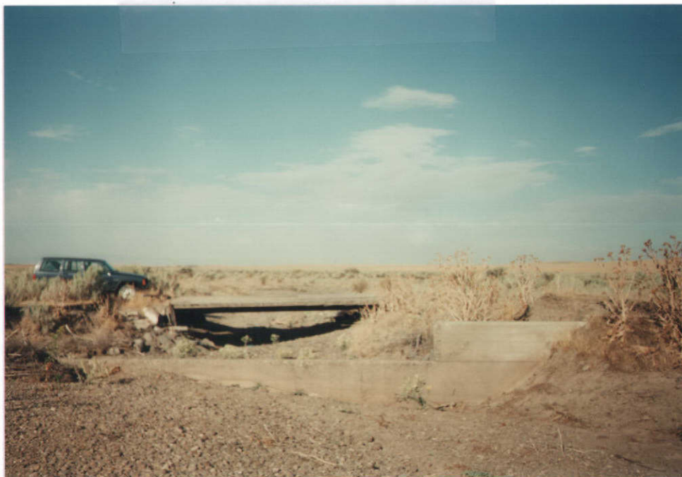
Photo #2 Looking DOWNSTREAM and SW from the same location as in Photo #1 showing a closeup of the concrete well. 9-12-96
