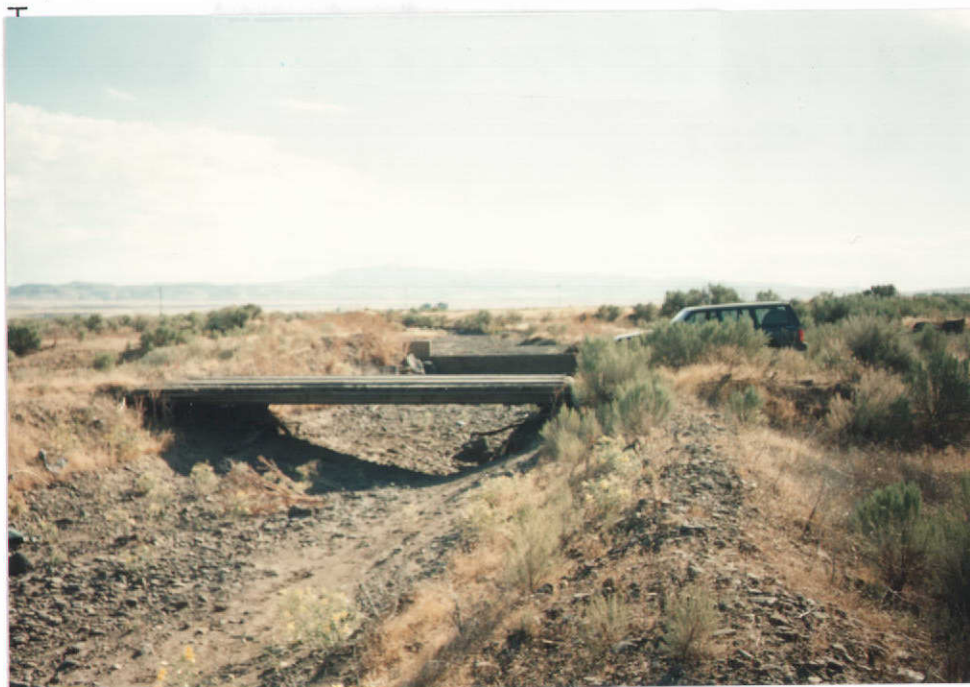
Photo #1 Looking NE UPSTREAM FROM the northern corner of T35 R6E Sec 10 NE SE NW showing a bridge & concrete well on canyon creek 9-12-96
