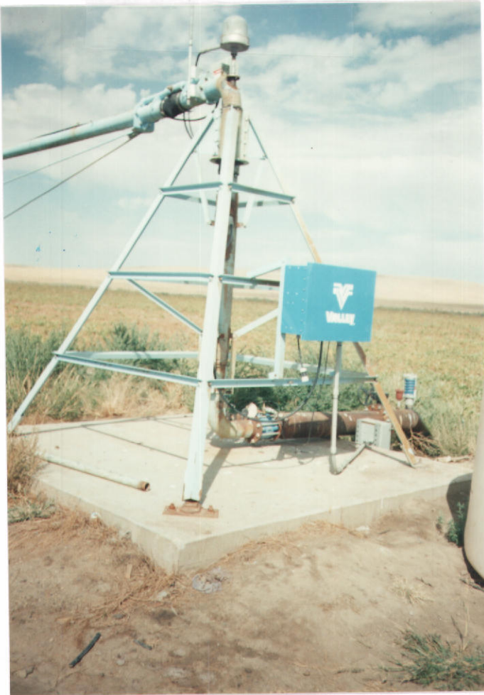
Photo #5 Looking NW From the SE NE of Sec 9 showing the East Pivot and the main line going underground to the North
