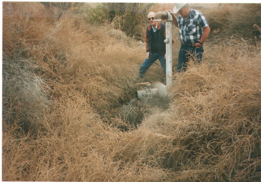
Facing east looking at the valve that has been opened to show some of the water discharged from the spring
