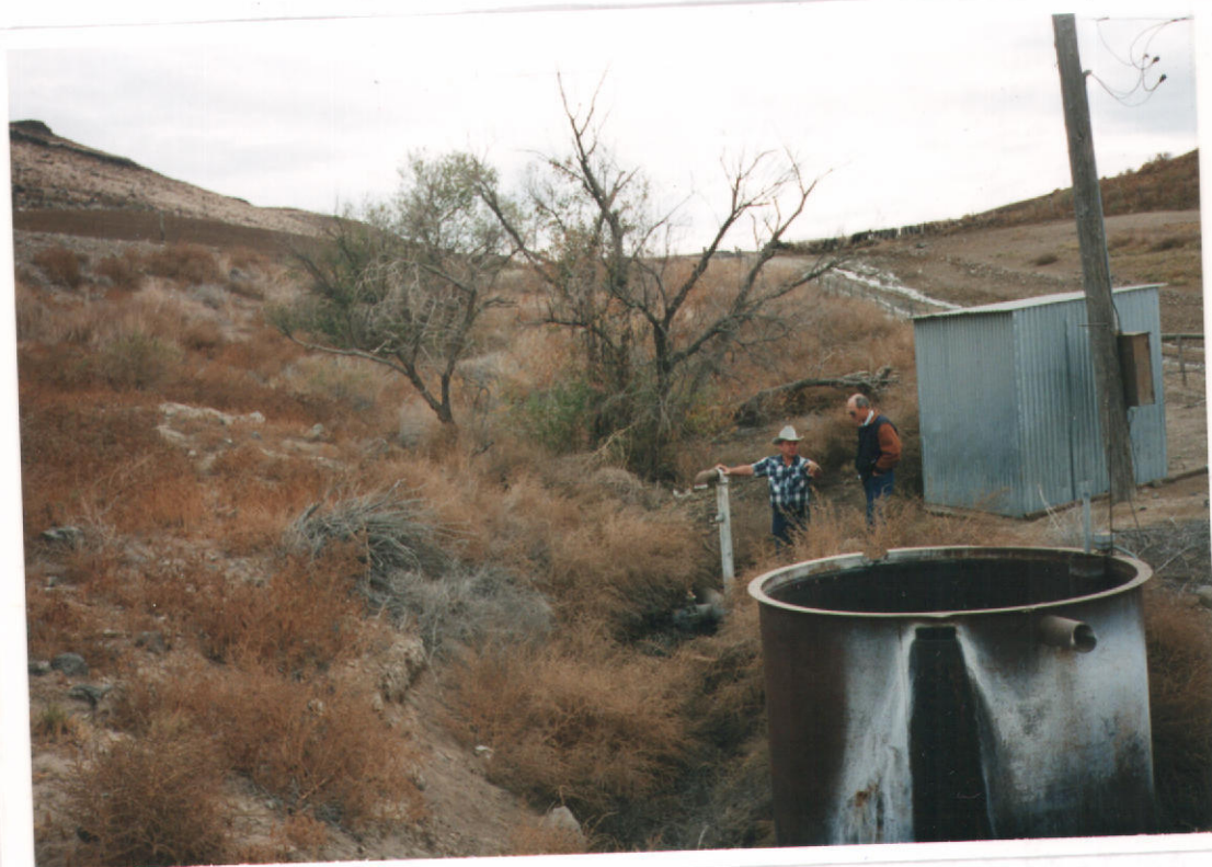
Facing east looking at the spring collection area. Standpipe to the right of center is for the overflow.
