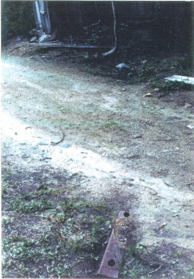
5. Culvert for Spring
