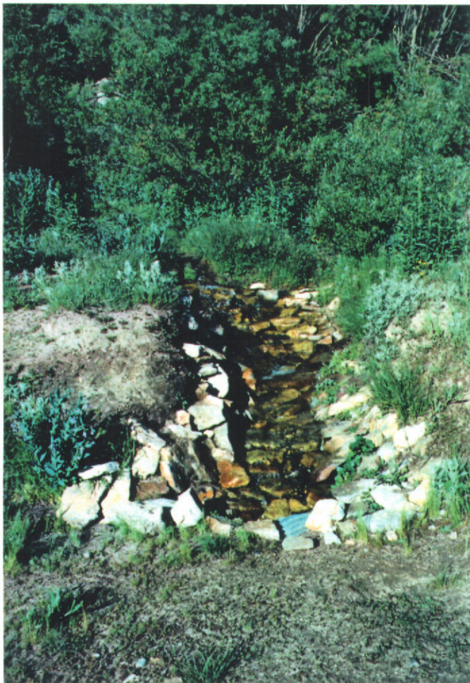
ROCK-LINED DITCH CHANNELS OVERFLOW (for location, see lower right in photo above)
