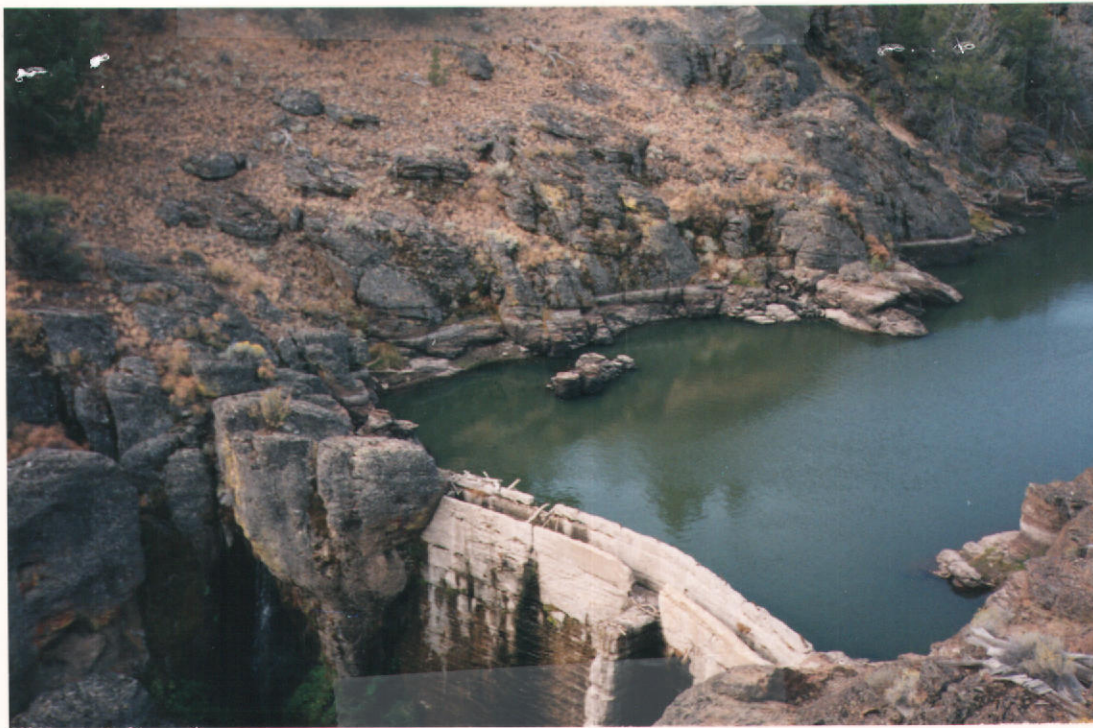
LOUISA CREEK DAM
