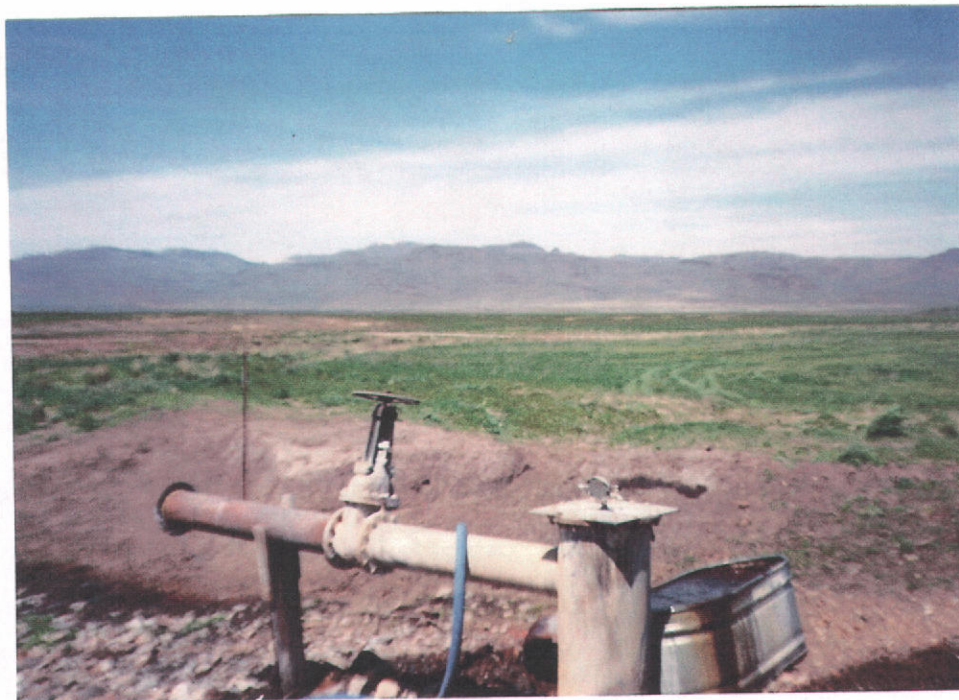
POD - "Two Plus" well - photo taken 4-30-96
