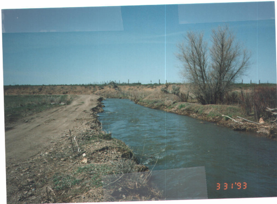
Diversion canal looking downstream from PID
