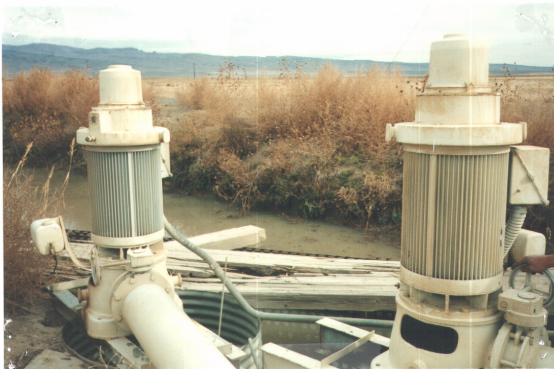
Pumping plant no. 1 on Bennett creek 2- 100 HP pumps
