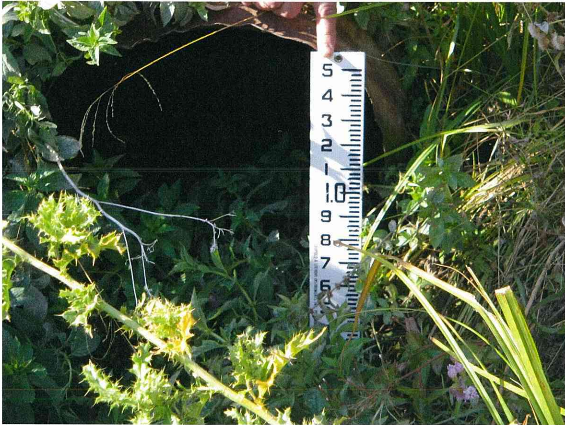
View showing scale of pipe where it empties into open ditch. Corrugated metal pipe was approximately 18 inches in diameter.
