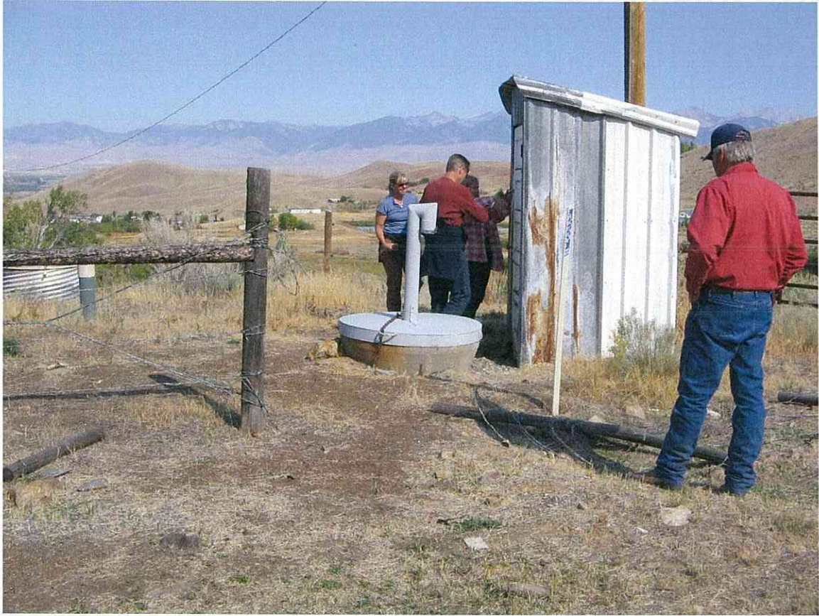
Outside view of pump house for 75-7032.
