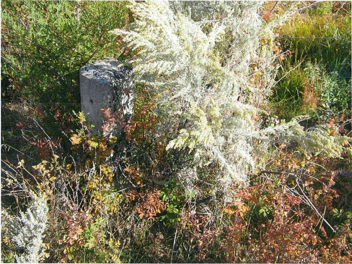
Photo taken showing concrete marker where water exits pipe system and enters open ditch. The open ditch then conveys the water to the North Fork Sevenmile Creek drainage.
