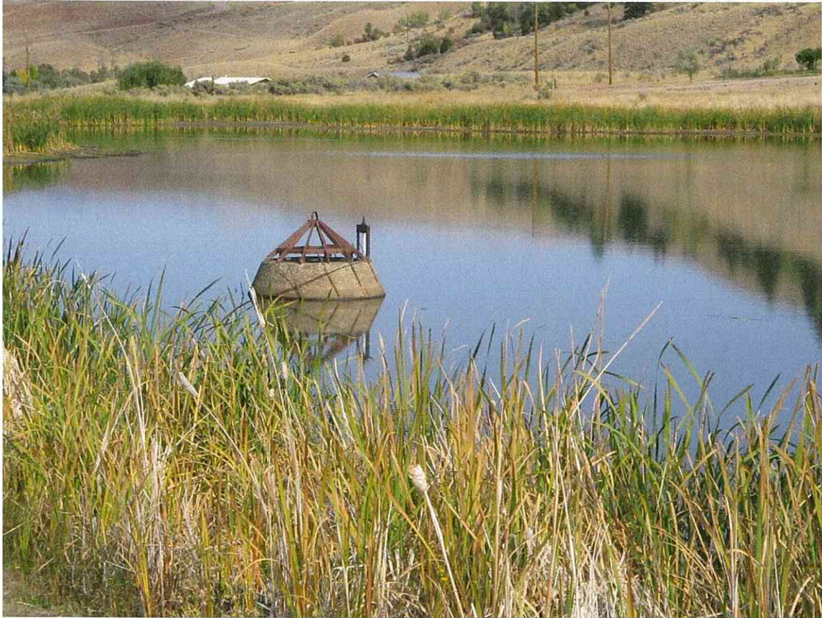
A view of the Hyde Creek Ranch point of diversion for Hyde Creek Ranch right 75-4395 from the pond seen in the last photograph. This photo was taken looking north/northeast. The water runs from this point of diversion under the dam and to the left of this picture. The photo was taken while standing on the dam for the pond.
