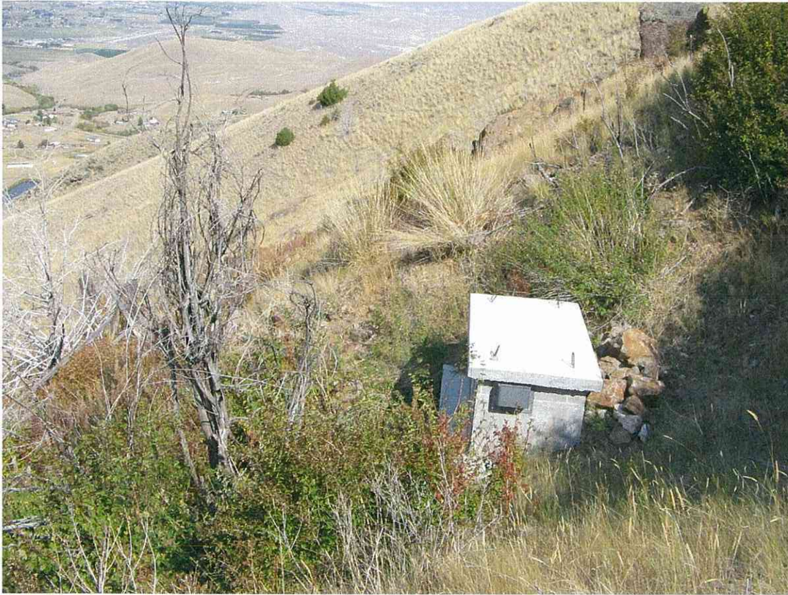
Outside view of spring box for 75-7032. A0017677.
