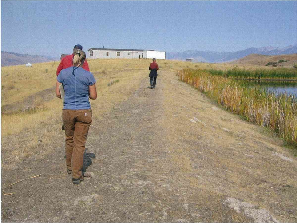
View of dam for pond. Hyde Creek Ranch point of diversion is out of sight to the right. The water runs through a pipe under the dam and empties into an open ditch to the left of this photo.
