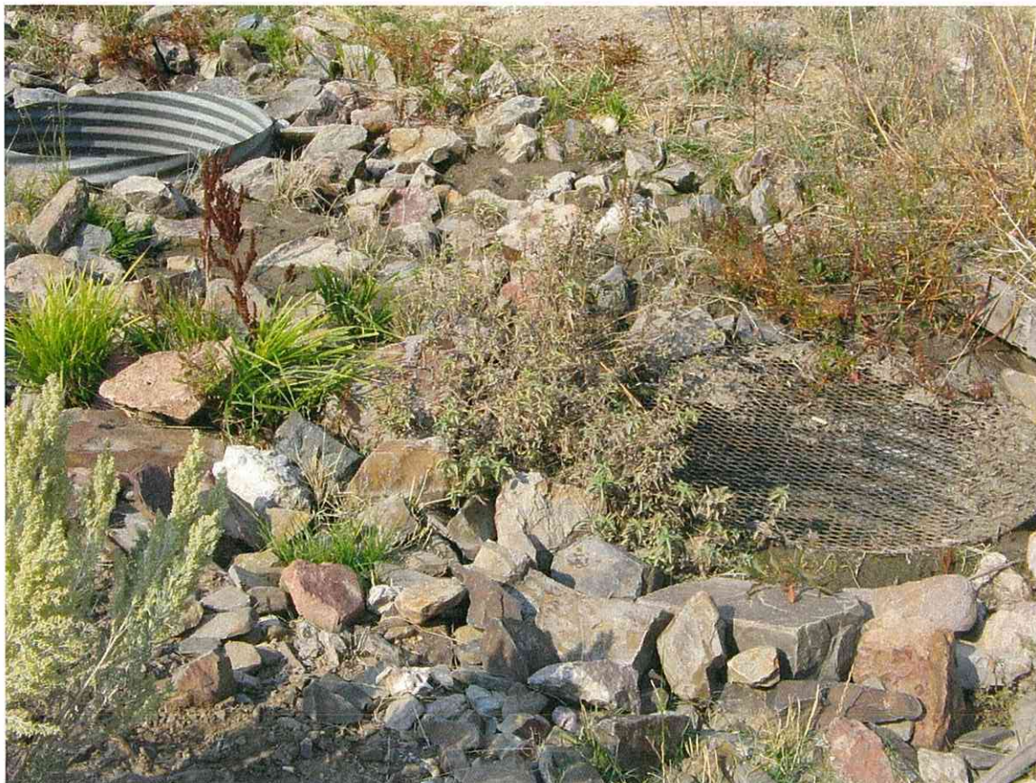
This photo is at approximately 20 feet above the elevation of Sunset Heights Water District's pump house. This photo shows the continuing conveyance for the Jackson property (75-14179) from South Fork Sevenmile Creek.
