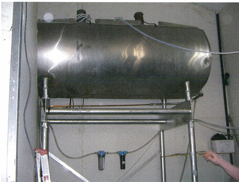
1200 gallon milk storage container used to store water and to send to bottling apparatus. The water from the spring is a constant 113 degrees F and, to be bottled, must be kept below 90 degrees. The milk storage container is double-walled and can be used to cool the water.
