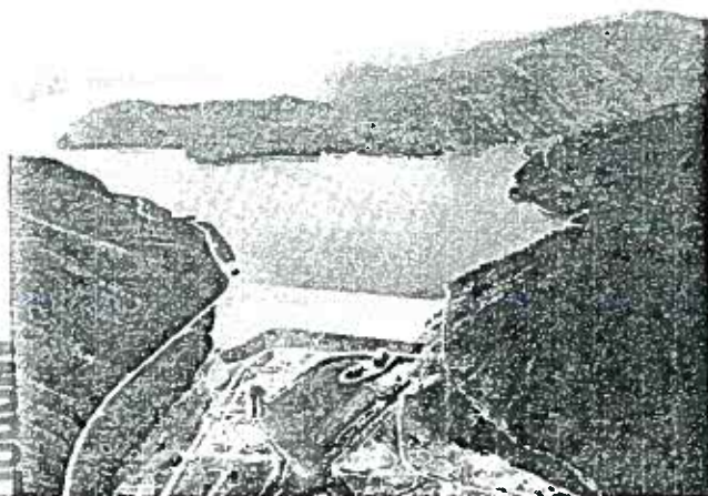
Palisades Dam and Reservoir
