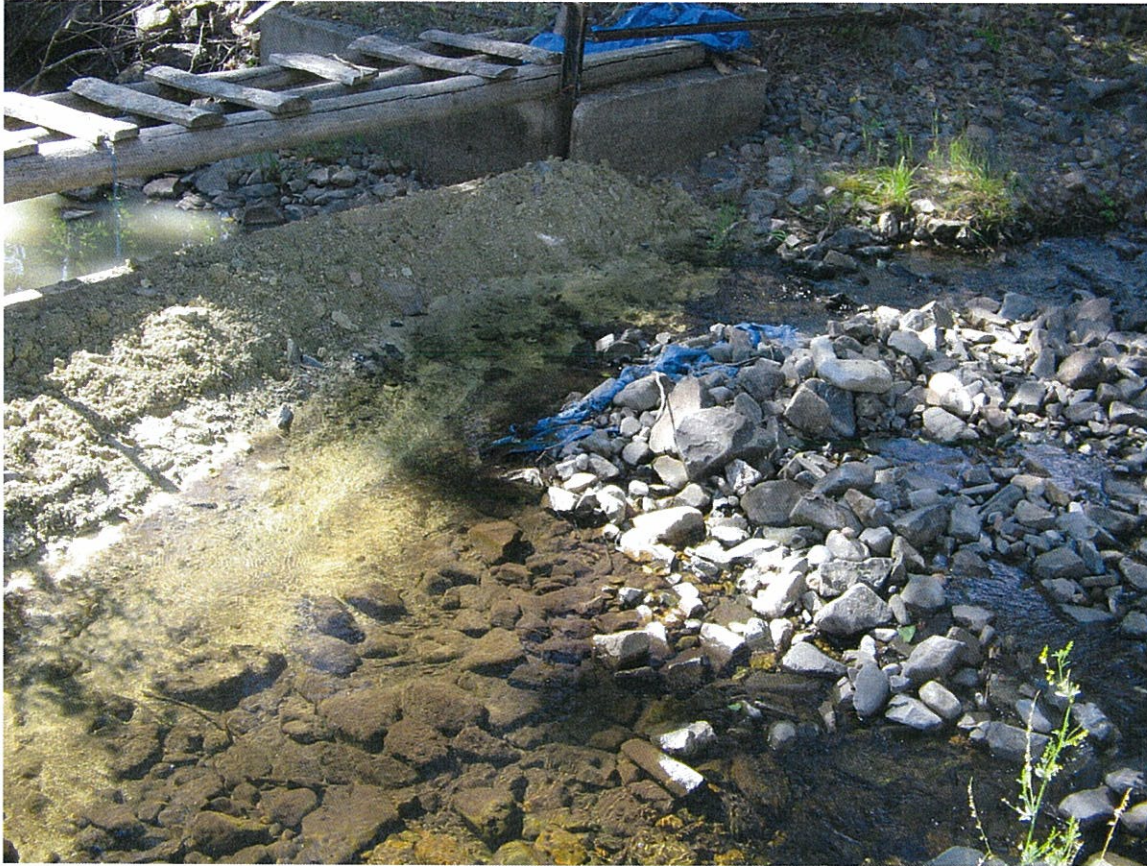
Photo of the lower part of the confluence of Jesse Creek and Pollard (Canyon) Creek. The headgate at the historic Jesse Creek channel can be seen here blocked with clay. Upstream is to the right and downstream to the left. The diversion for Farmers Ditch is slightly behind and to the left of the vantage point of the picture. This picture was taken while facing south and slightly east.
