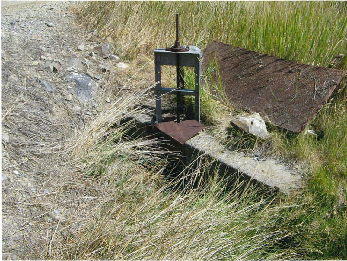
Photo of a headgate along the lower ditch (right-hand ditch of the previous picture). Beyond this point, the ditch is piped and serves the Lois Blackadar/Jim Juza property. Upstream is to the right and slightly behind the viewer. Downstream and down-valley is leading away to the left of the viewer.
