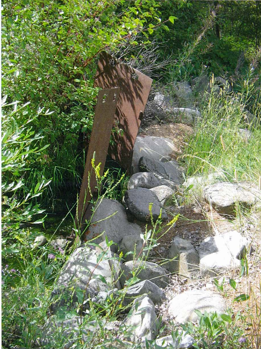
Photo shows the two intakes for Arrowhead Water Dist's rights. The intake in the background is the intake for Arrowhead's domestic rights. The water goes through a small culvert into a gravel trough where it is filtered, and then travels into Arrowhead's piped domestic system. The foreground diversion is for Arrowhead's irrigation rights, which are then distributed through its reservoir system.
