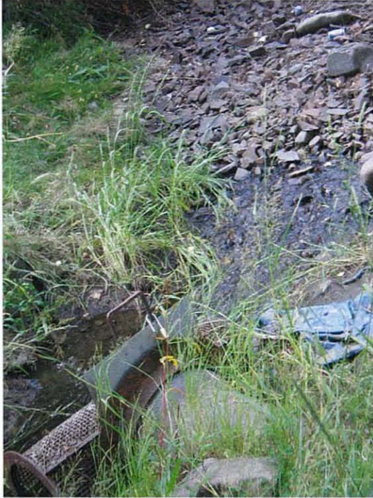
Photo showing Arrowhead's Pollard Creek ditch where it enters pipe. Arrowhead's outlet from reservoir (shown previous picture) is just to the left of this picture.
