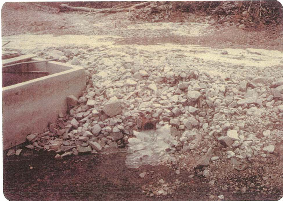
Photo #2. Outlet of Chipps Creek pipeline just above the Pollard Canyon water intake. This flow from Chipps Creek augments the Pollard Canyon flow.
