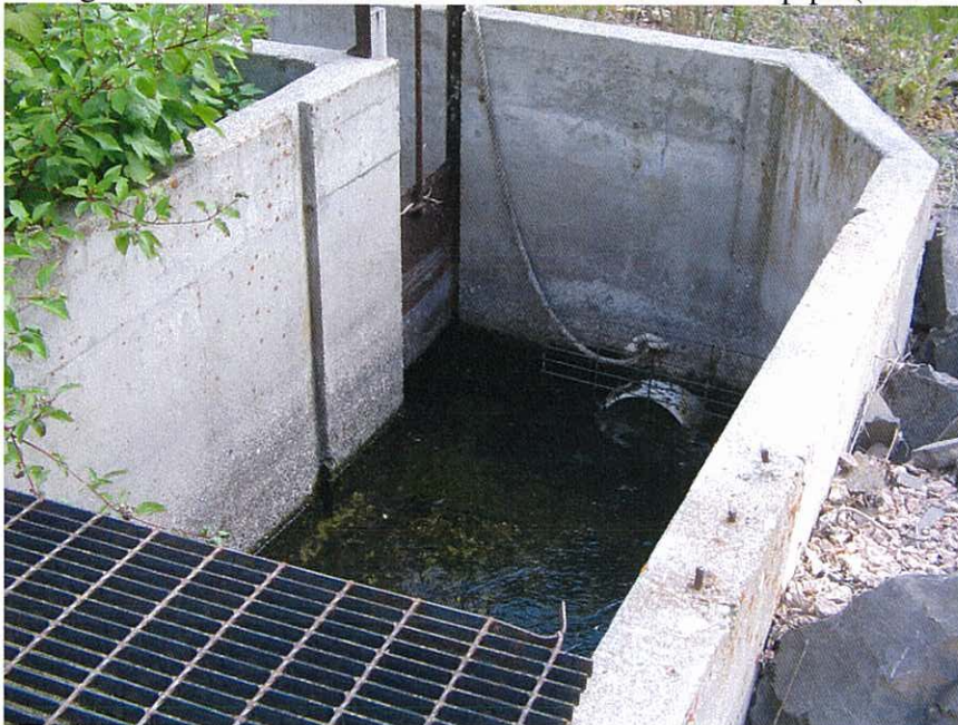
This picture was taken by turning right from the vantage point of the previous picture. Water would flow from the wire mesh at the diversion point and into the white pipe seen in the right-center of the picture. That pipe then flows down and dumps into Jesse Creek above the City of Salmon's Jesse Creek diversion. The metal headgate seen to the left-center is used to release any excess flow.
