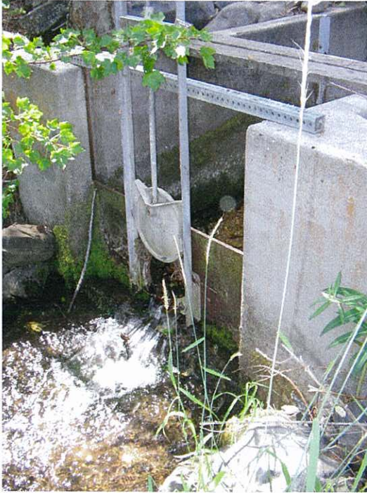
Photo of Chipps Creek headgate. The City of Salmon diversion is just upstream of this site, approximately 4 feet.
