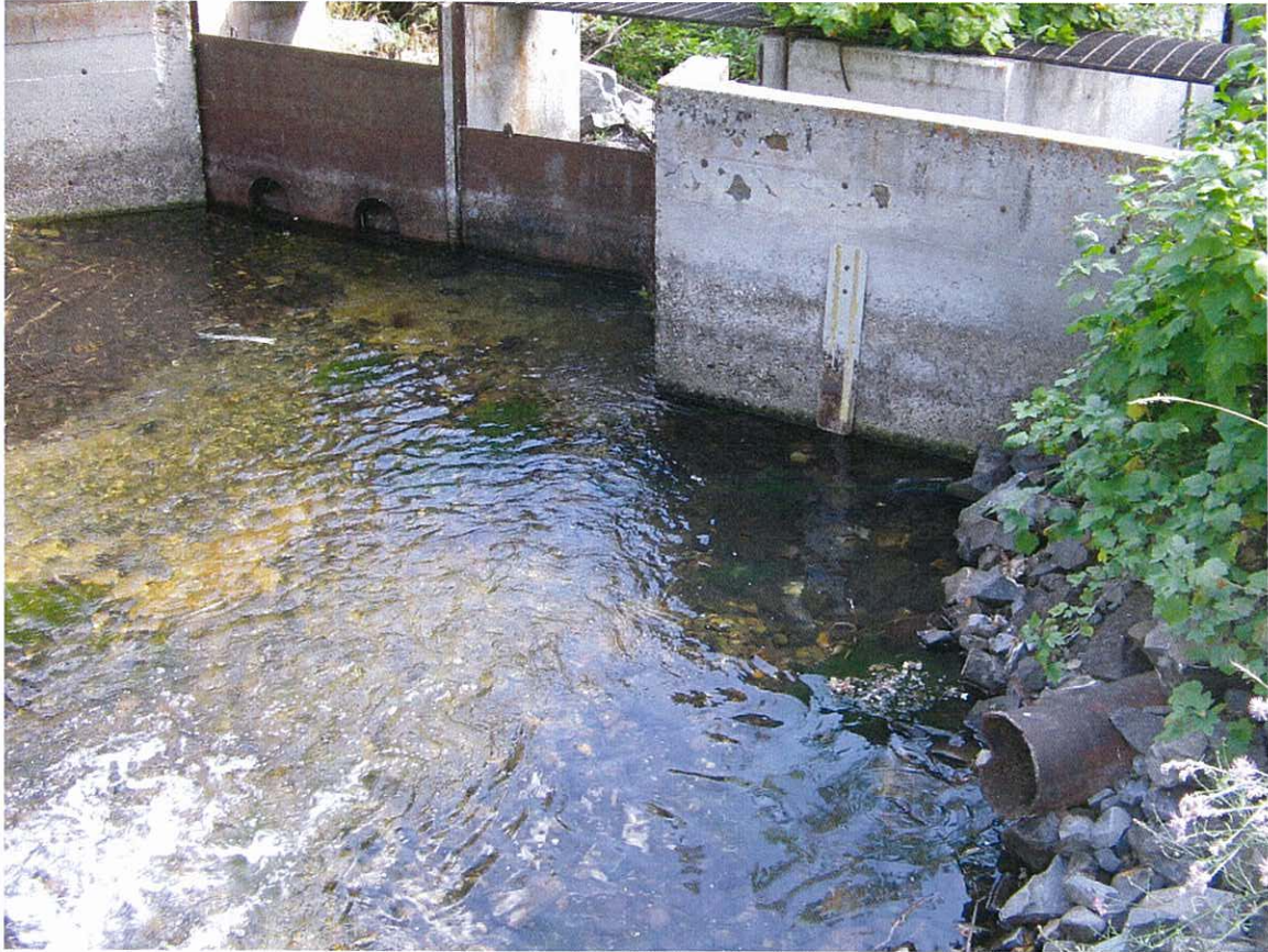
To the right foreground in this photo, the pipe from the City of Salmon's Chipps Creek diversion can be seen. That pipe dumps into Pollard Creek at this point. The City of Salmon's Pollard Creek diversion is just behind the cement wall in the center of the photo. The two metal gates in the left-center of the picture are opened to allow the un-diverted flow down the main channel.
