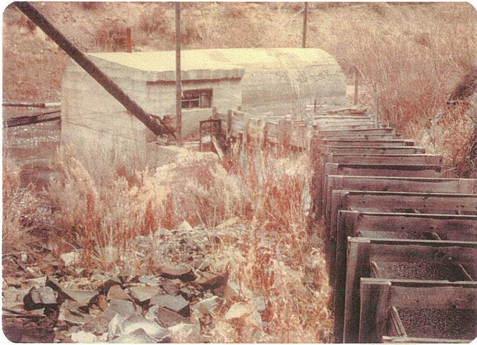
Photo #5. Wood flume in Jesse Creek. The concrete structure is the Jesse Creek water intake.
