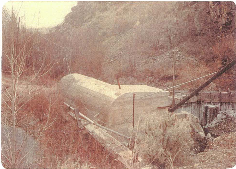
Photo #6. Jesse Creek water intake. Wood flume on right carries Jesse Creek flow. The large black pipe carries water from Pollard Canyon. Near bottom center of photo is a well the City uses to augment the water supply.
