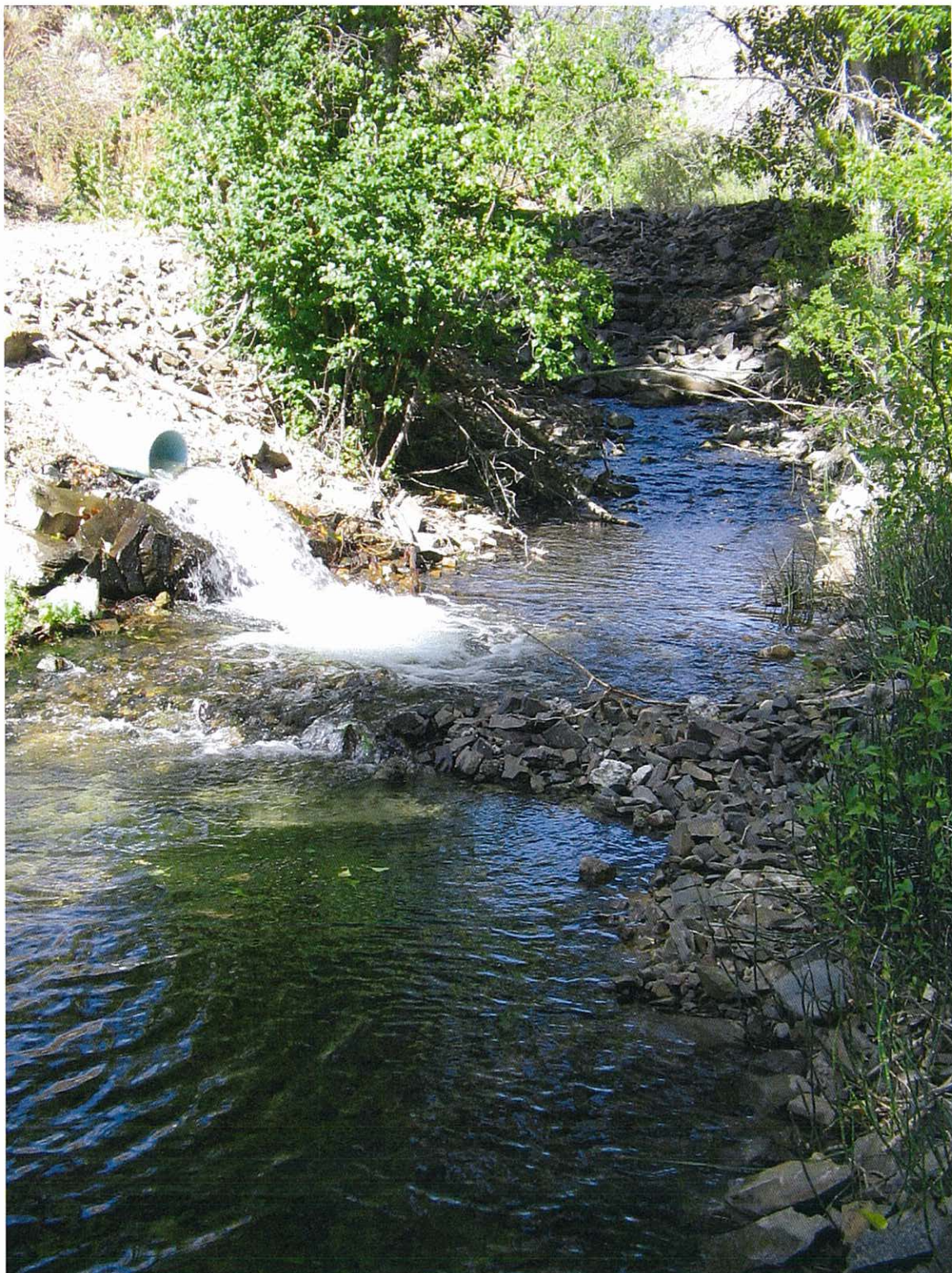
Another view of the Pollard Creek pipe pouring into Jesse Creek. This photo was taken from downstream near the City of Salmon's Jesse Creek diversion.
