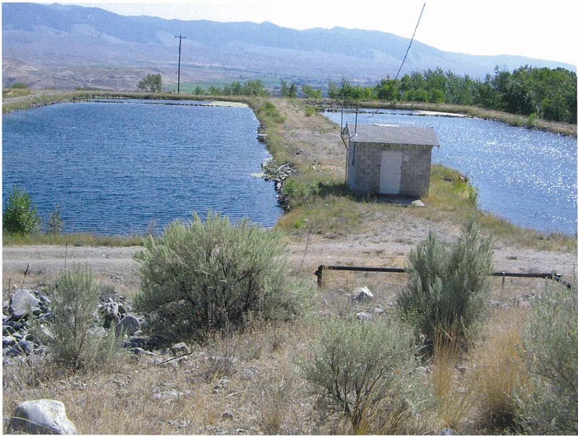
View of the current two active settling ponds for the City of Salmon treatment plant. The water for the system runs underground from Jesse Creek to the building in the right-center where it is divided between the two ponds. The radio antenna seen on the left background side of the building signals the Salmon River pumps if supply gets low so the City can then pump from the Salmon River to augment their supply.
