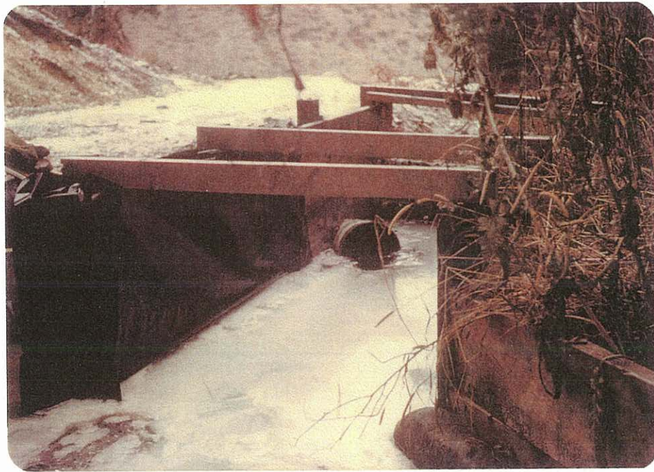
Photo #1. Chipps Creek water intake. The 12 inch pipe carries water to augment the Pollard Canyon flow. This facility is on private land.
