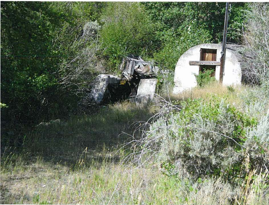
An additional view from downstream of the old City of Salmon waterworks. The Jesse Creek channel runs from the area of the pipe seen in the center towards the left edge of the picture.
