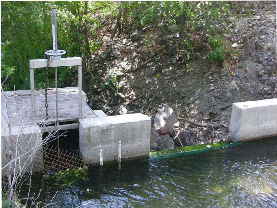
View from upstream of the City of Salmon's Jesse Creek point of diversion. The actual point of diversion can be seen in the left-center behind the tree with the wire mesh placed in front of the opening. Jesse Creek's natural flow continues in the right-center of the picture.
