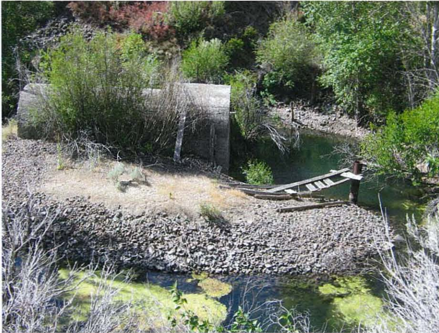
This is a view of the old City of Salmon waterworks on Jesse Creek. These waterworks were put in place sometime after the City of Salmon bought the Salmon City Water Company and before 1974 when the current system was installed. The right of the picture is the upstream side. Jesse Creek runs in the background of the picture and is not visible here. The water seen standing in this picture is most likely seepage from the Jesse Creek channel.
