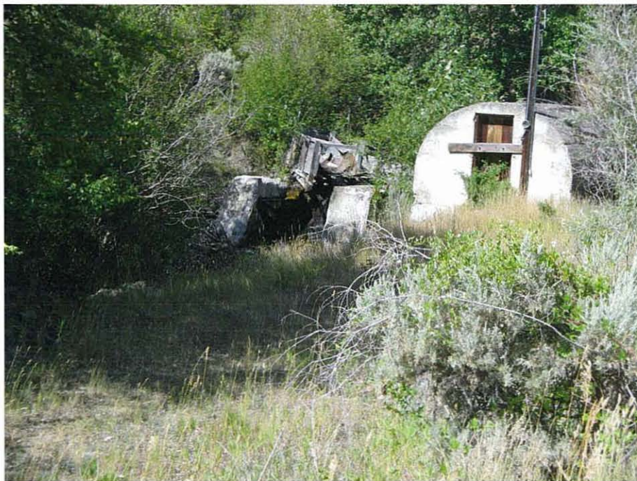
An additional view from downstream of the old City of Salmon waterworks. The Jesse Creek channel runs from the area of the pipe seen in the center towards the left edge of the picture.
