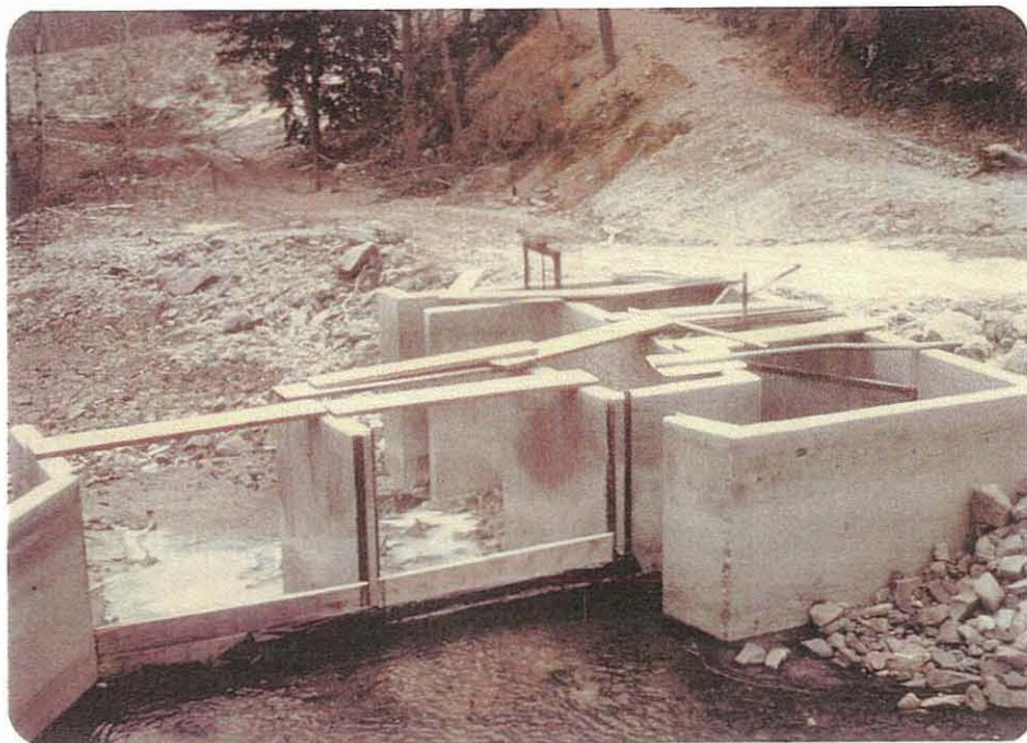
Photo #3. Pollard Canyon water intake. A buried 12 inch pipeline carries water from here to the Jesse Creek water intake.
