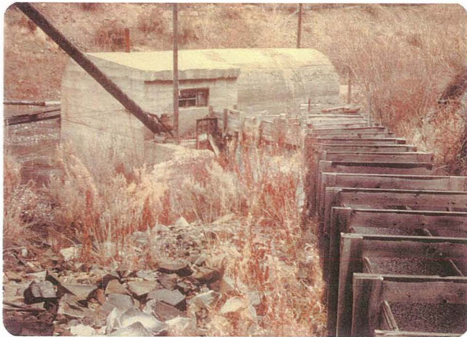
Photo #5. Wood flume in Jesse Creek. The concrete structure is the Jesse Creek water intake.
