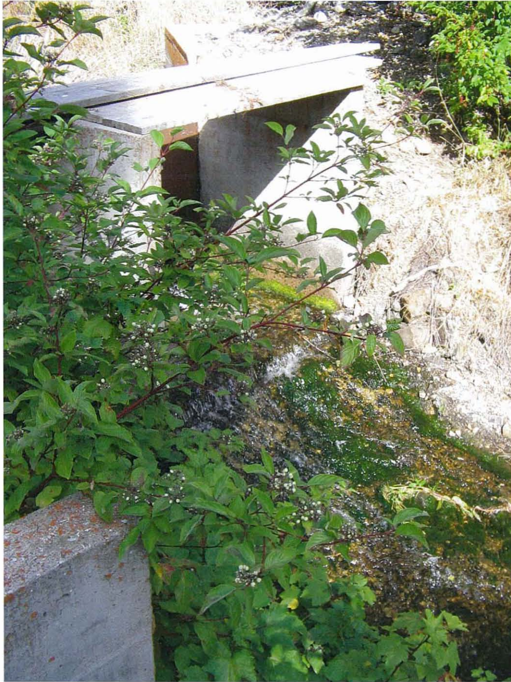
Photo showing the downstream end of the City of Salmon Pollard Creek diversion. The headgate to release excess flow is invisible behind the brush in the far left portion of the picture. The water seen flowing here is the Pollard Creek water that bypasses the point of diversion.
