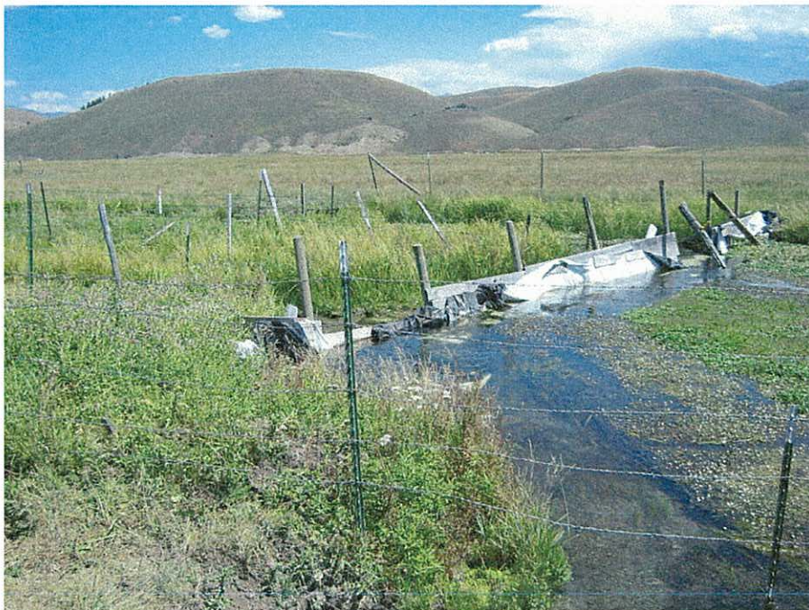
POD (2738543-x 1289804-y) facing east (07S 46E S33 SE SE NW).
