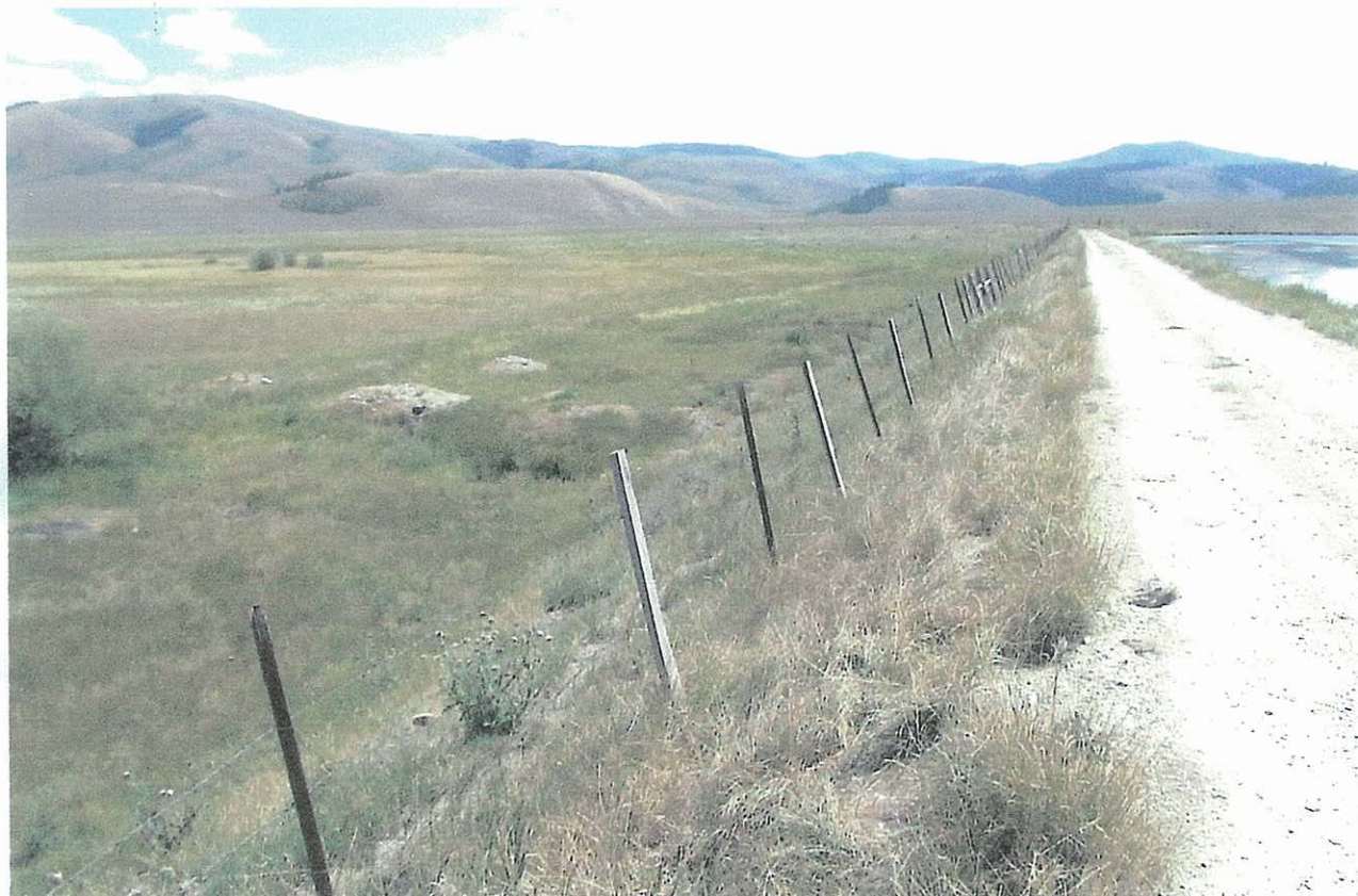
Right side downstream slope.
